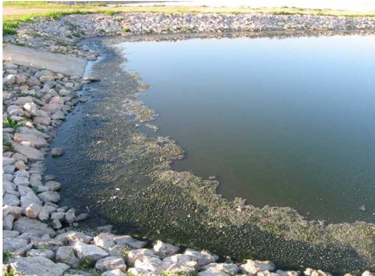
Fig. 3.6: Shallow lagoons for wastewater settling
