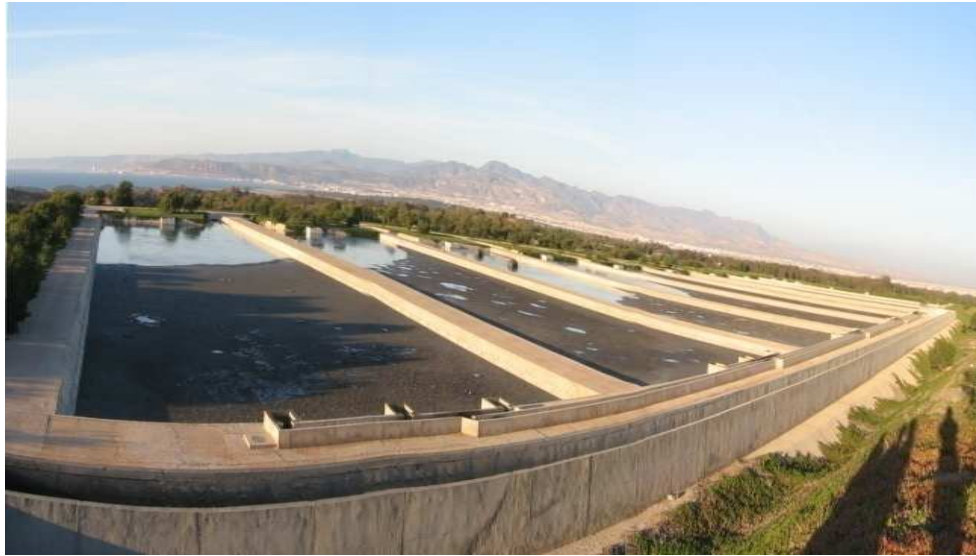
Fig. 3.3 Wastewater treatment plant near Agadir
