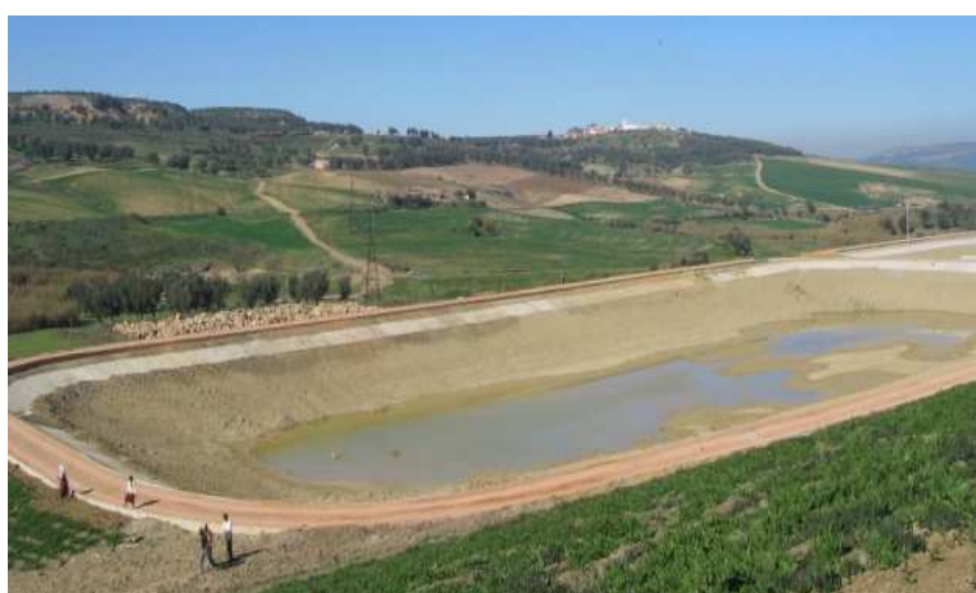
Fig. 3.2 Meknes treatment plant
