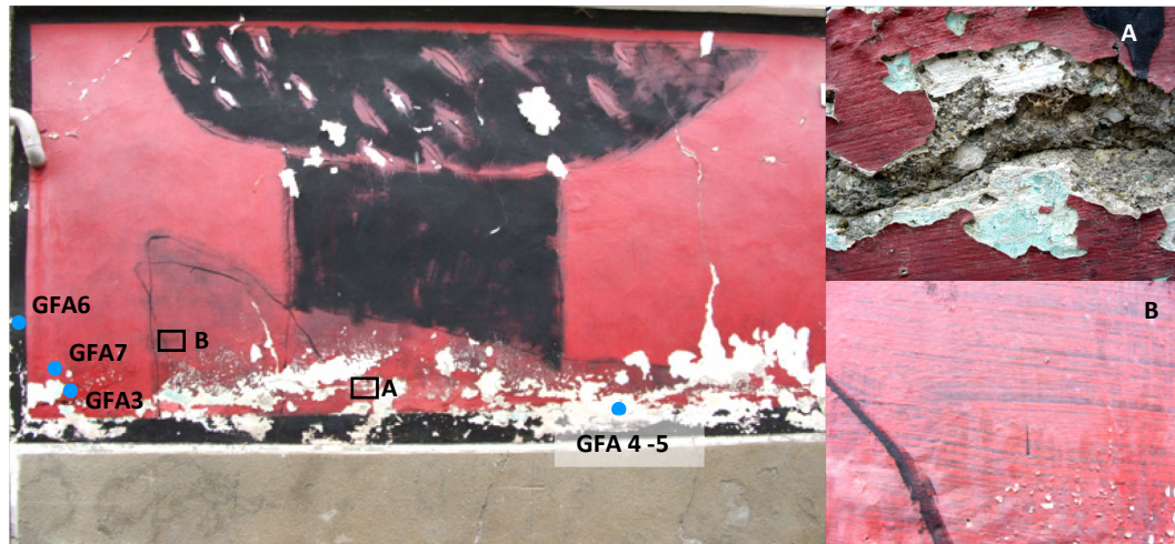
Fig. 4.1-4: Asveri's mural as it looks today. A and B: enlarged details documenting the condition of the mural. The blue dots mark the sampling points.
