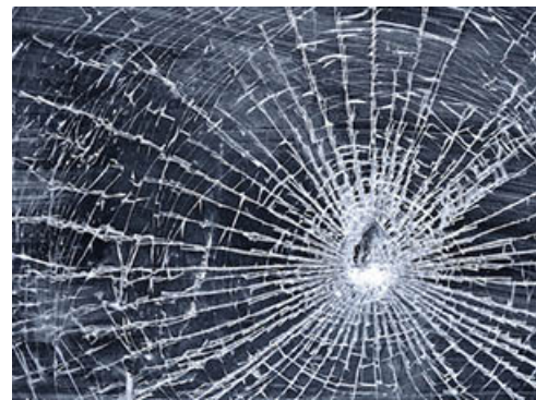
(b) Broken glass.
