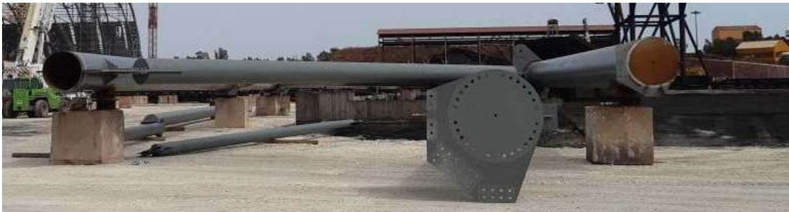
Figure 29. Beams with CHS section before installation
