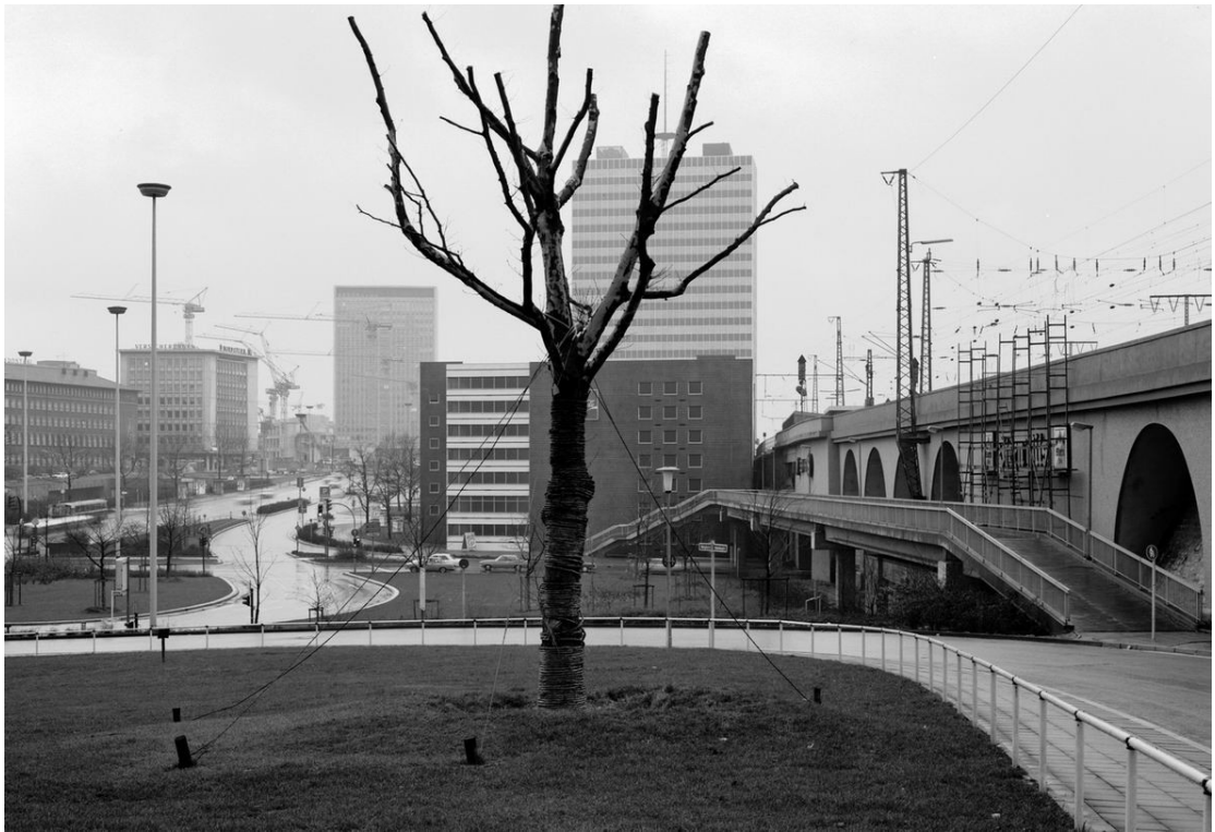
45. Essen-City, Gildehof-Tunnel, Hauptbahnhof, 1976.
